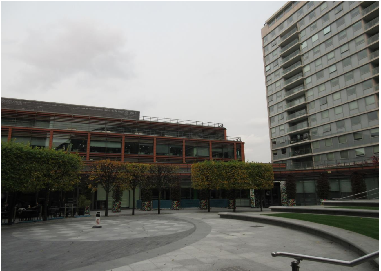
12 Cardinal Walk South elevation from roof top garden
